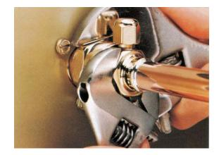
It is important that ONLY the nut on the pre-charged tube be turned, or the diaphragms will be torn out by the piercing knives and they will be loose in the refrigeration system. Note: As the couplings are tightened, the diaphragms in the quick connect couplings will begin to be pierced. As that happens, there will be some resistance to tightening the swivel nut.
